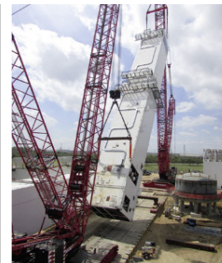
Coldbox erection for a SCALE 60 plant in Texas, USA.
