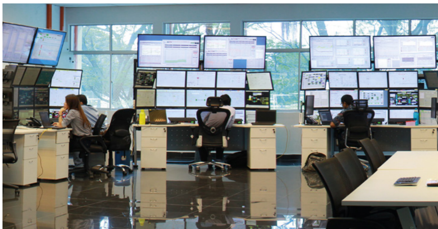
Remote Operating Centre (ROC).
