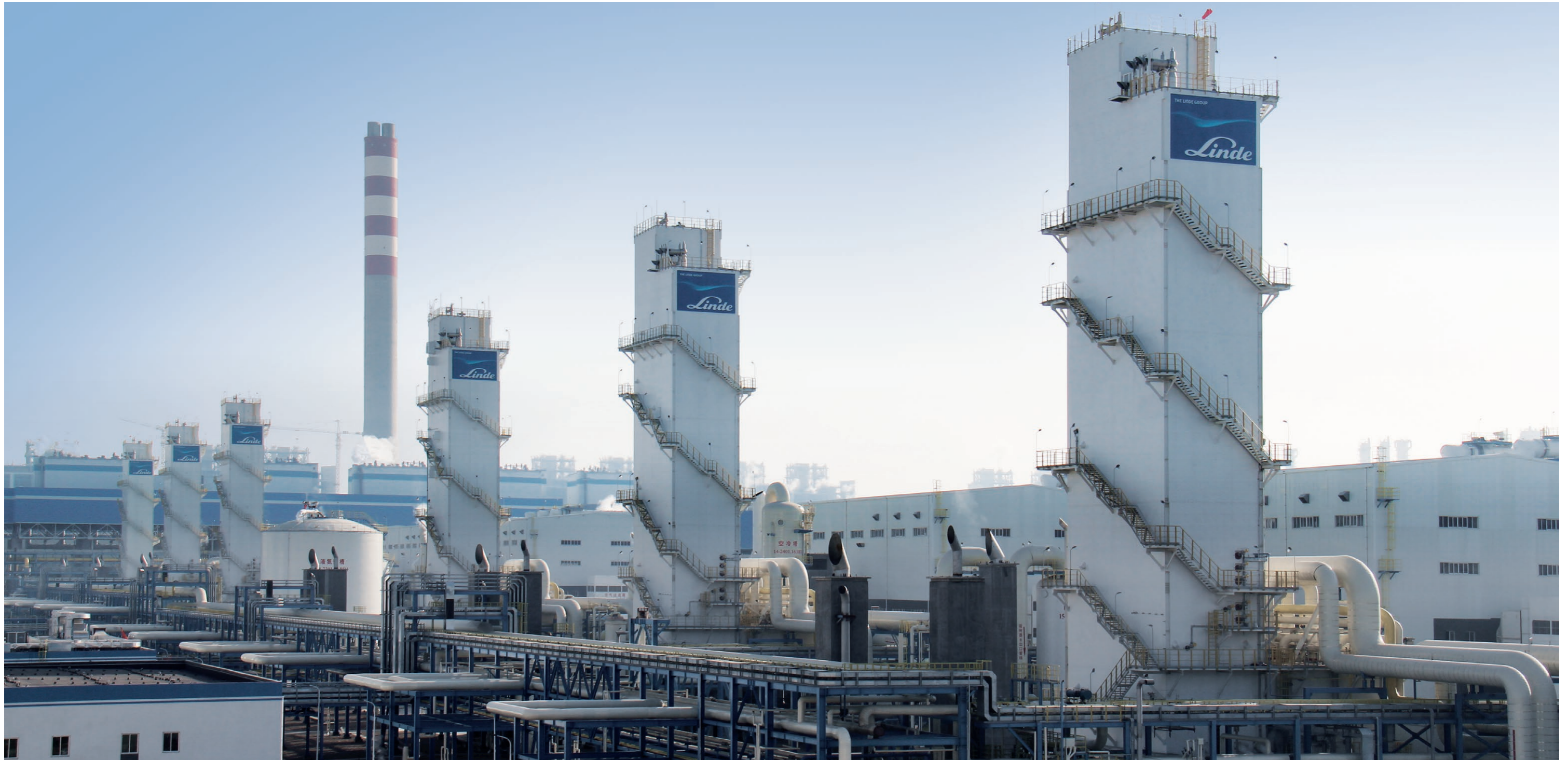
Air separation units near Yinchuan City, China.
