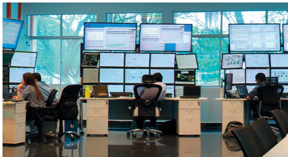
Remote Operating Centre (ROC).
