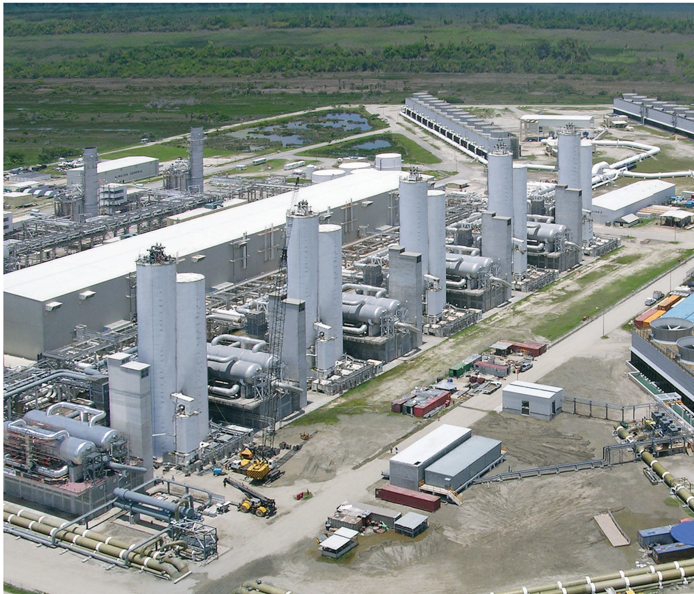
Air separation units at Cantarell, Mexico.
