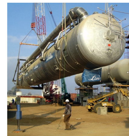
Lifting of a column.
